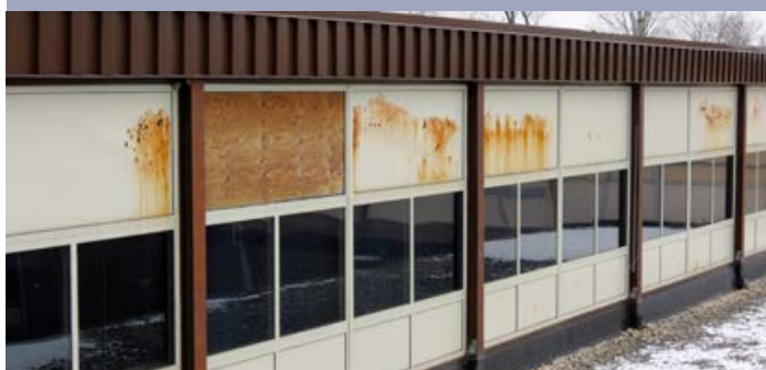
Original Windows and Failing Exterior Panels
