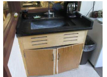
Leaky sinks & peeling casework
