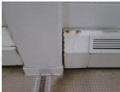
Deteriorating vents & floor
