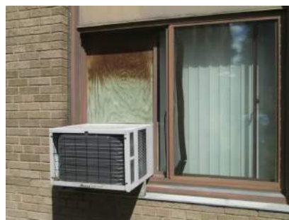
Leaking A/C units & windows
