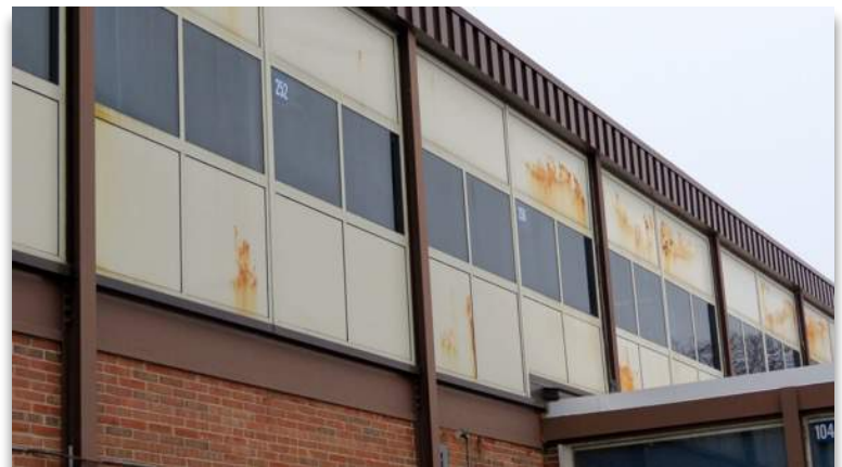
Exterior walls along the the high school are rusting and deteriorating.
