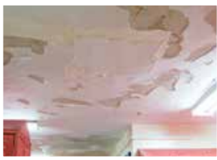
The ceiling structures in several MTSD school buildings are in need of repair
