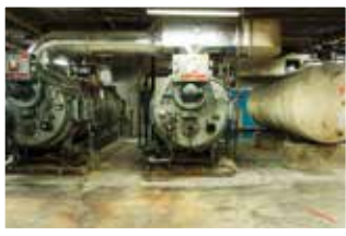
The boilers in most of MTSD's school buildings are 30-50 years old
